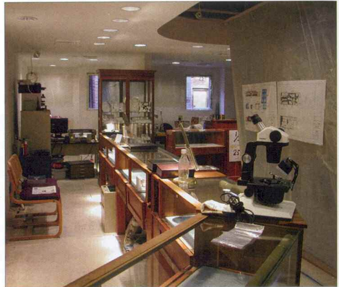
DURING. At Summerwind Jewelers in Portsmouth, NH, a remodeling project presents obstacles to the daily routine.
