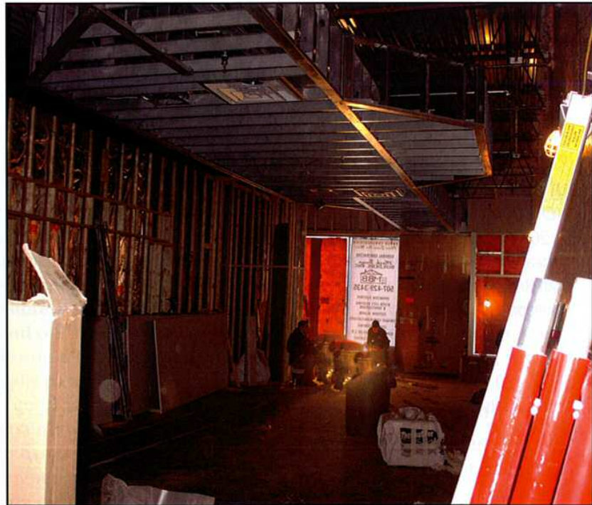
The second half of the store under construction. Display windows at front of store are papered over.
