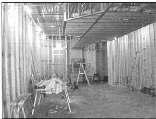
Walls were taken back to concrete and studs.
